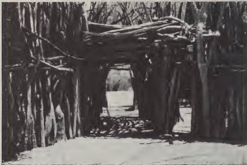
Fig. IV. Close-up of Gateway showing details of construction and "wicket gate"
