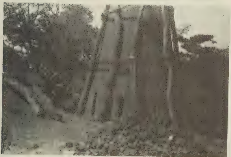
Kiln with heap of ironstone in the foreground—Draught pipes in background.
