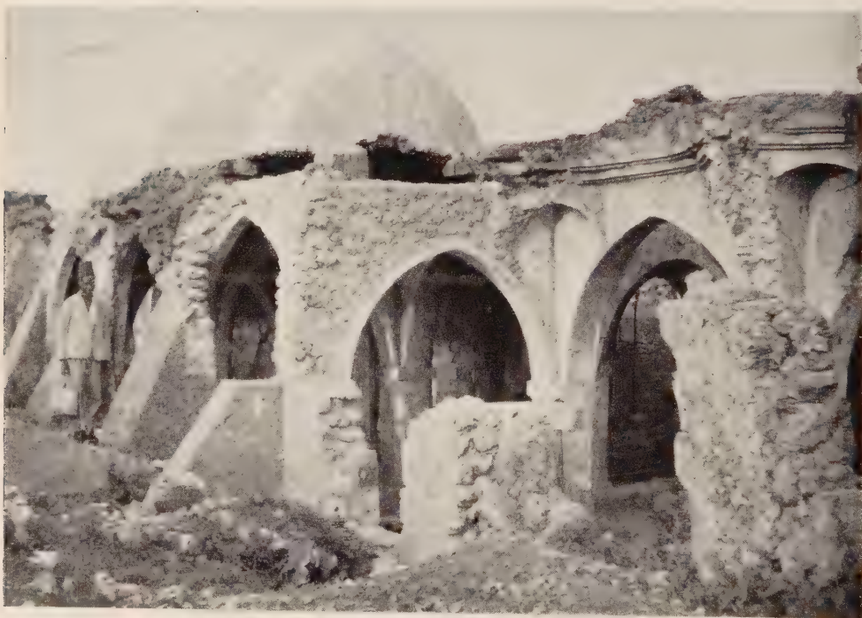
Plate IV. Part of the Great Mosque, Kilwa Kisiwani, during reconstruction.
