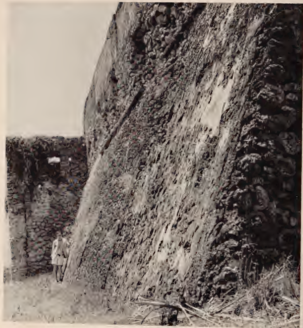
[Courtesy Public Relations Department] Plate III. The battered wall on the north side of the Palace.
