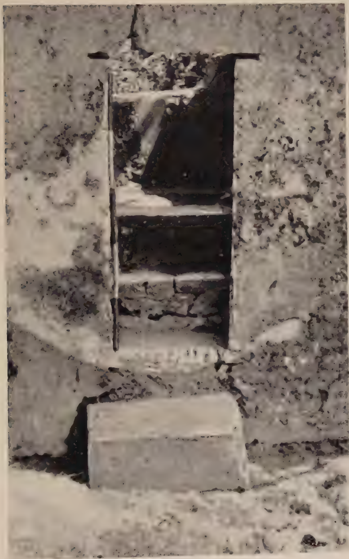
Plate IIa. Access to Circular Tower.
