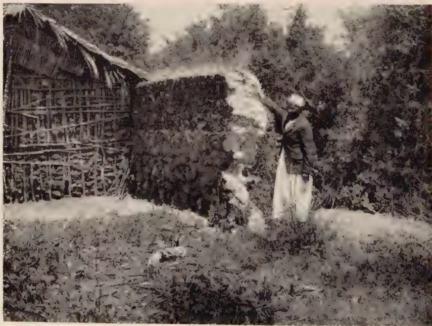
Fig. II. —Wall at Zingibari undermined by tidal action, shows also house built against the wall.
