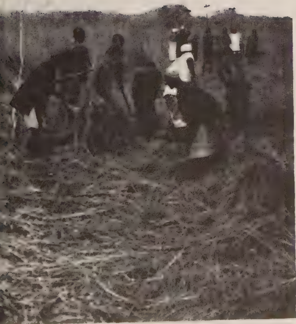
The great Lukaya Swamp, over two miles wide, was a formidable obstacle. Once the ground was fairly dry the grass, shoulder high, was first flattened, then cut up with hoes and, when dry, burned
