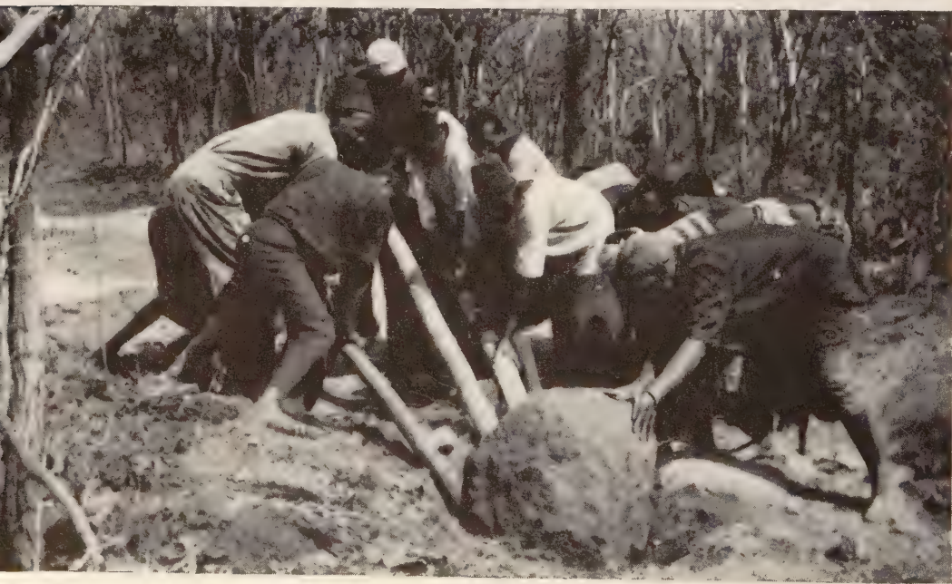
Before evacuation could begin hundreds of miles of roads had to be constructed
