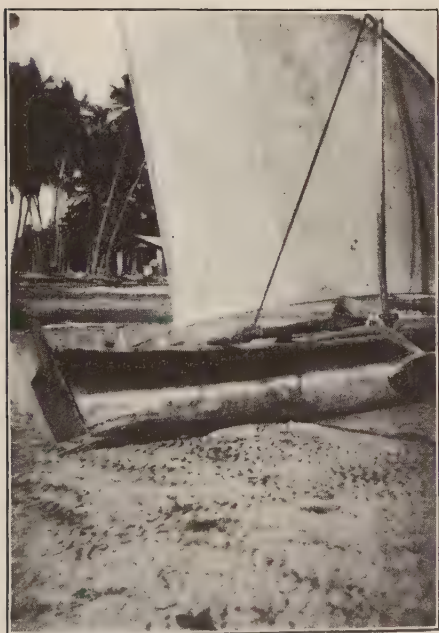
Fig. 3.—Close view for details of Rigging, mrengu and ndulu (stem). The chipi is clearly shown
