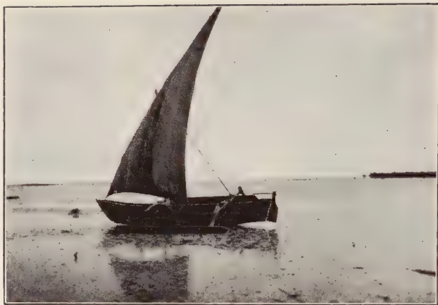
Fig. 2.—General view from Leeward. The rail is in position for running across wind; the demani is passed round the stem of the leeward ndubi
